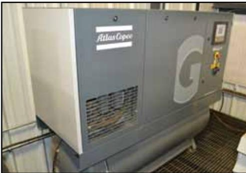
**ATLAS COPCO GA22 30-HP Rotary Air Compressor**
