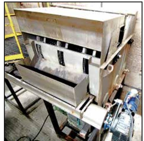
HYCOR SS ROTARY DISC FILTER, SYSTEM #2
