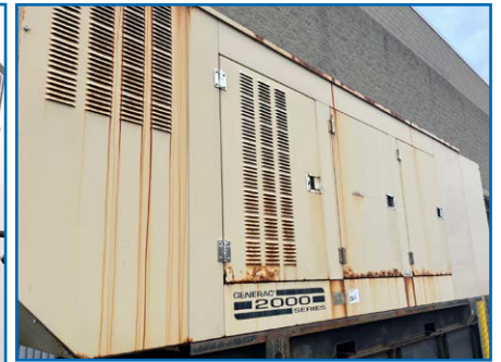
GENERAC 2000 SERIES DIESEL BACKUP GENERATOR
