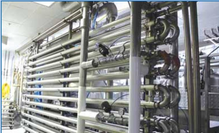
WAUKESHA CB 12-PASS SS TUBE IN TUBE PASTEURIZER
