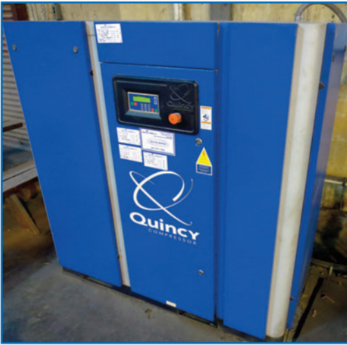
QUINCY 30HP ROTARY SCREW AIR COMPRESSOR WITH DRYER
