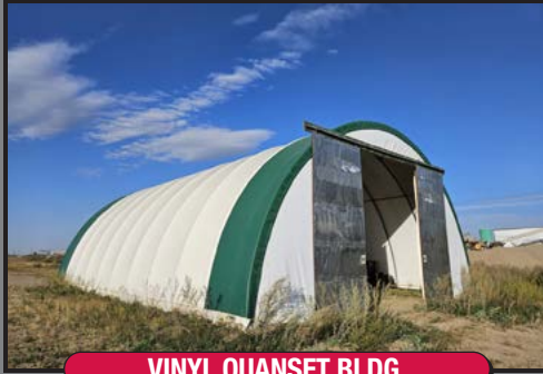
VINYL QUANSET BLDG.
