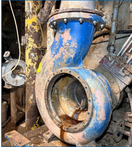
PARTIAL VIEW OF GOULDS CENTRIFUGAL PUMPS
