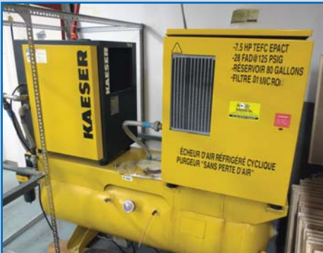
2004 KAESER 7.5HP Rotary Screw Air Compressor And Air Dryer Mounted On Horizontal Tank s/n 1320
