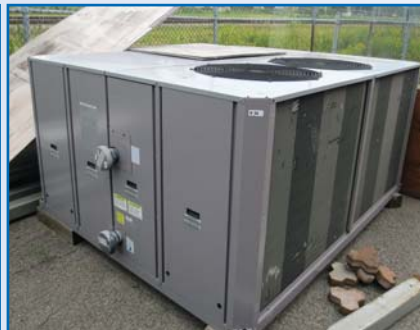
CARRIER 30RAN035 Chiller With Fans
