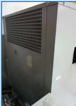
BEMAG 550KVA Transformer
