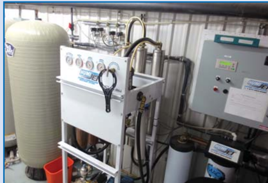
HUMIJET Spray Humidification System With SIEMENS TD200 Control With Reserve Tanks, Controls Etc.
