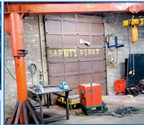
PARTIAL VIEW OF JIB CRANES
