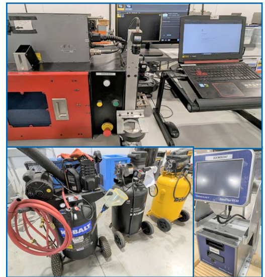
PARTIAL VIEW OF SUPPORT EQUIPMENT
